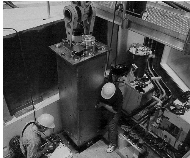
Fig. 150. Photograph of one of the 5 modules, the beam entrance module, being lowered into the west target station.
